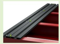
STEP 10: Repeat until the deck is complete, cutting the last board to width to fit if required
