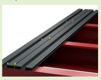
STEP 10: Repeat until the deck is complete, cutting the last board to width to fit if required
