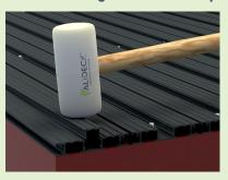
Important note: you may need to cut the last board to width to fit, if so please ensure to not cut into the central fixing channel as this will compromise the integrity of the decking board.
